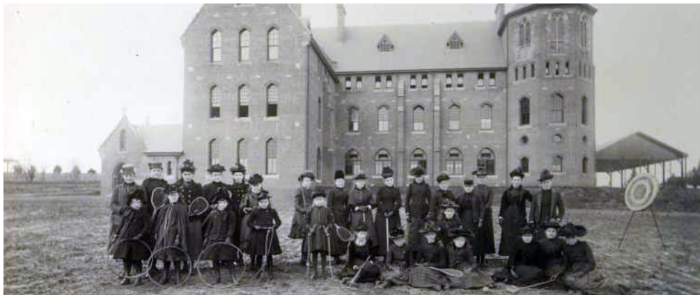
Genazzano College, founded in 1889. The property in Kew was originally secured as an all-girls' boarding school by the twelve founding Sisters who had set sail from England in 1882, to help meet the growing need for Catholic Education in Australia. Together with William Wardell, an eminent colonial architect, they oversaw the construction of the stunning Wardell Building in 1889, and in April 1891 the Sisters and their pupils took possession of their new College.
